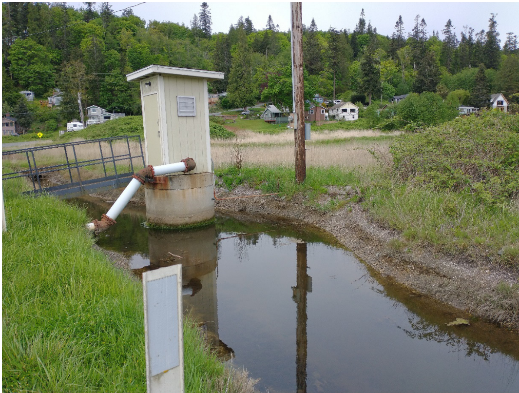
Photograph 4 – Pumphouse and Adjacent Drainage Ditches Looking West
