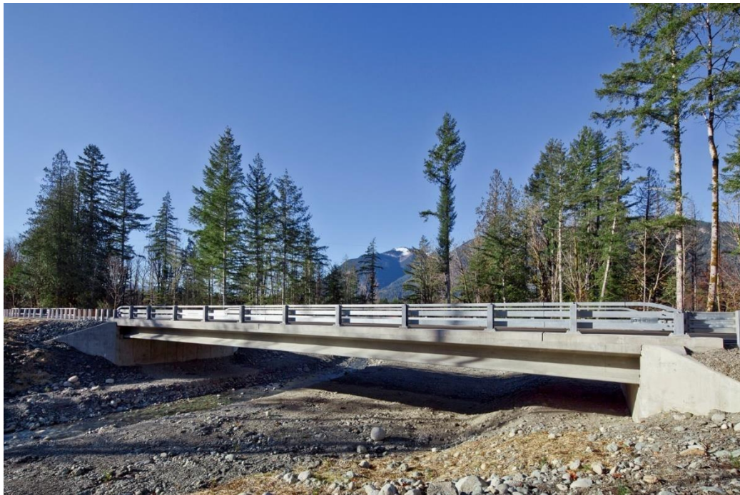
Figure 5-1: Illabot Creek Bridge
