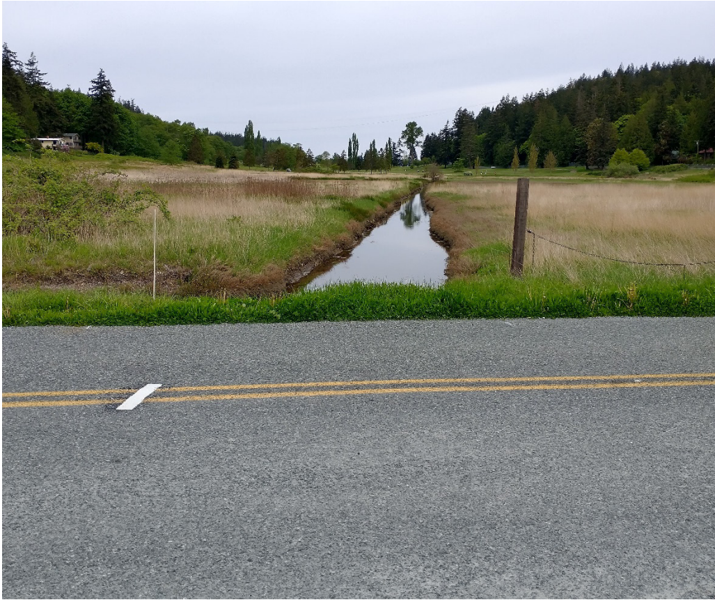
Photograph 3 – Central Drainage Ditch Looking North Across Satterlee Road
