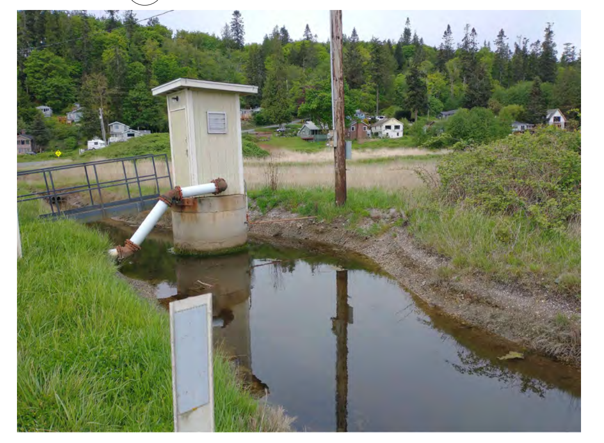
4 PUMPHOUSE - VIEW WEST
