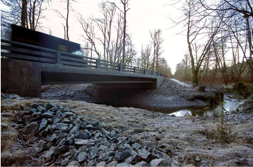
Figure 6-1: Davis Slough Bridge
